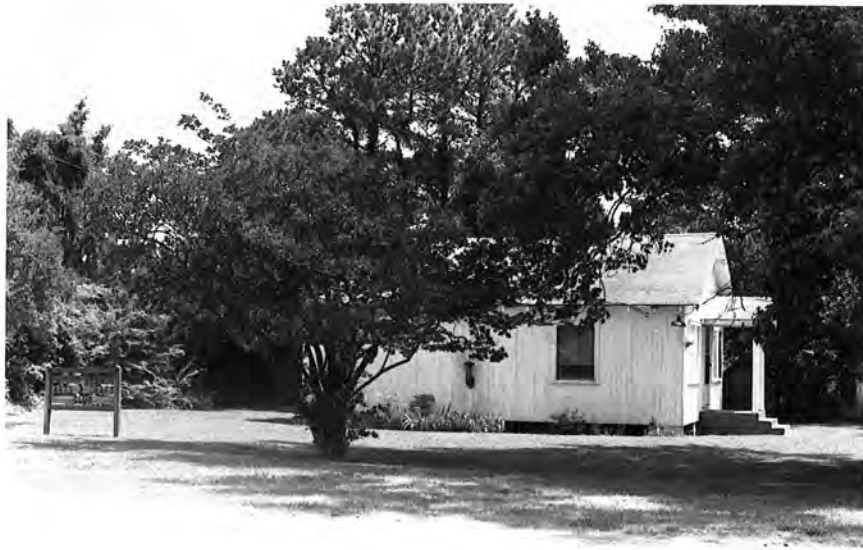
Plate 53. Poplar Branch Arts and Crafts Center - West Elevation and Porch
