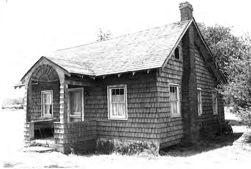
Plate 43. Daniel Saunders House - Facade
