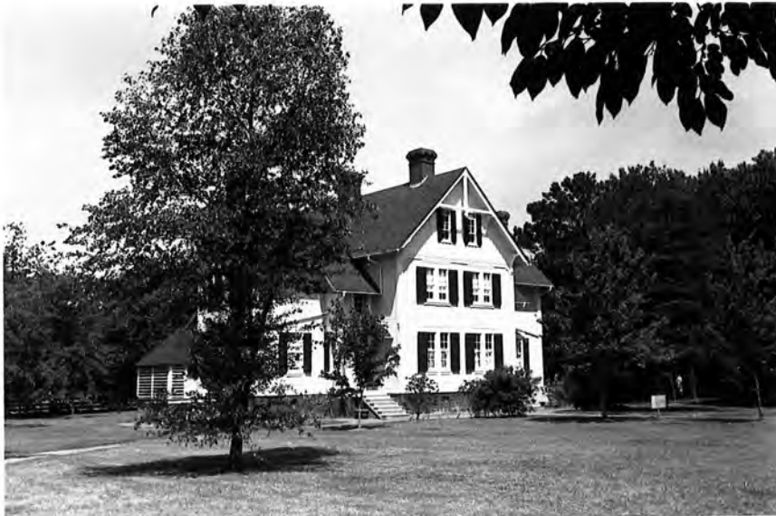
Plate 2. Currituck Beach Light Station, Keeper's Cottage, Looking North.
