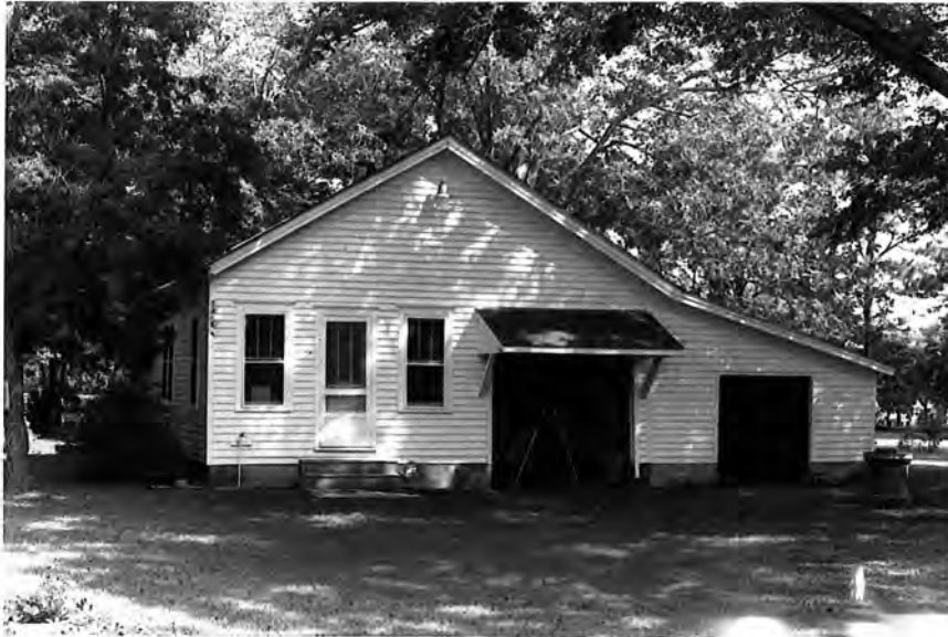
Plate 29. Dr. W.T. Griggs House - Office/Garage
