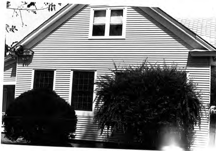
Plate 51. (Former) Gallop School - South Elevation
