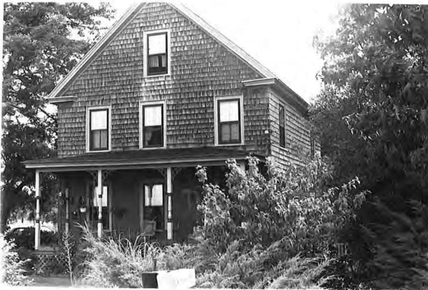
Plate 36. Currituck Sound Rural Historic District - Bromsey House
